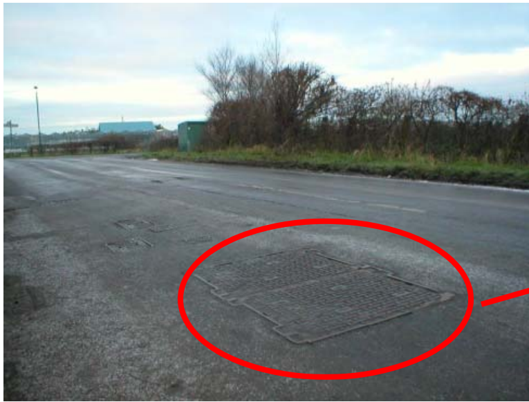
Manhole covers in a UK road. (Southport)
