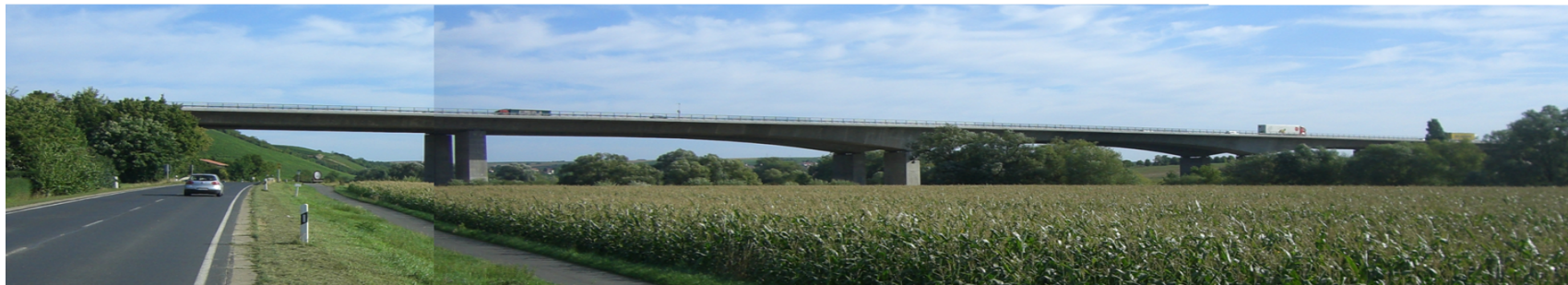
Test installation in a bridge (359m long in Bayern)
